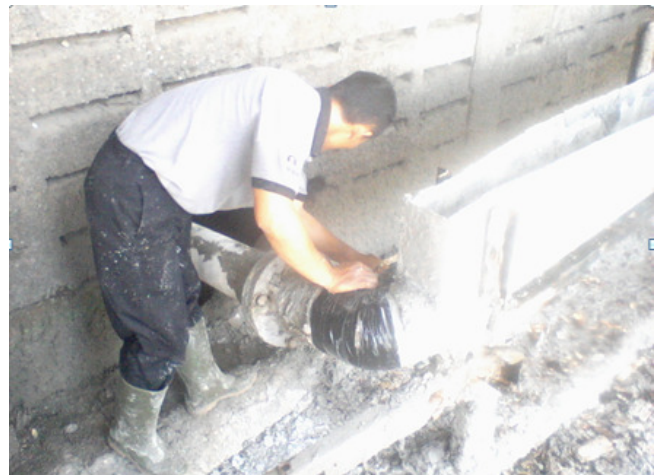
Leaky input feed pipe.
